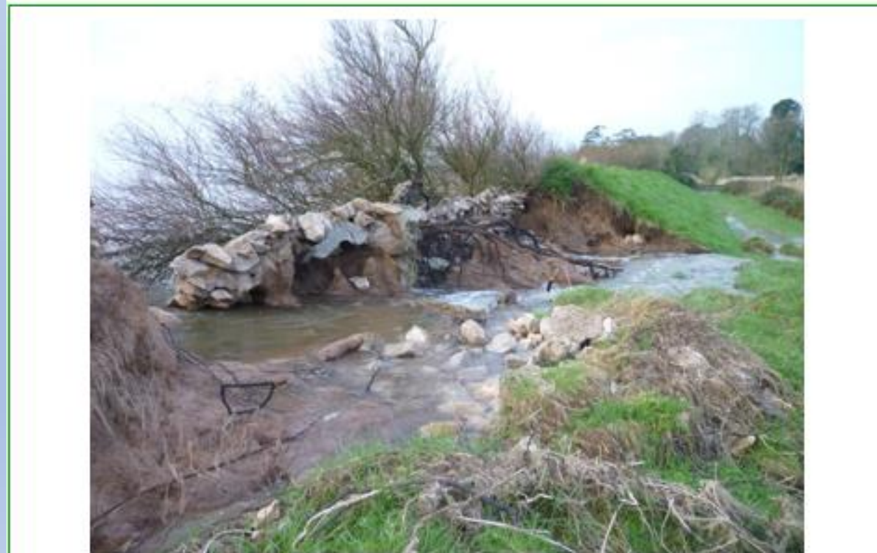
Figure 4: Photo of 2014 Breach of flood bank
